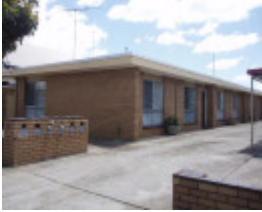
29 Glenleith Avenue, Drumcondra
