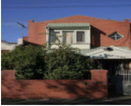
CREMORNE WELLINGTON STREET 47 Unit 1.jpg
