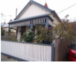
RICHMOND BENSON STREET 7.jpg
