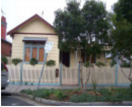
RICHMOND BELL STREET 2.jpg
