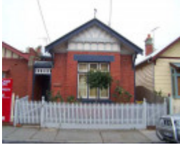
RICHMOND BELL STREET 4.jpg
