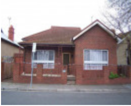
RICHMOND BELL STREET 10.jpg
