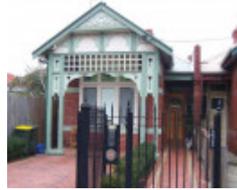
RICHMOND BELL STREET 15.jpg
