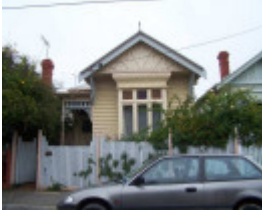
RICHMOND BELL STREET 16.jpg
