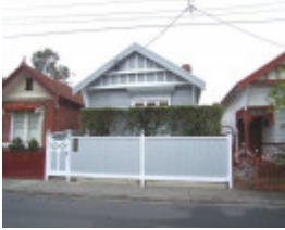
RICHMOND BELL STREET 20.jpg
