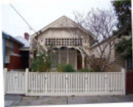
RICHMOND BELL STREET 21.jpg
