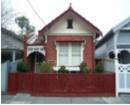
RICHMOND BELL STREET 22.jpg
