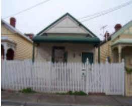
RICHMOND BELL STREET 27.jpg
