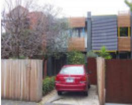
RICHMOND WALL STREET 2-4 Unit 3.jpg
