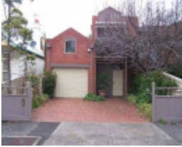
RICHMOND WALL STREET 6.jpg
