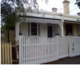
RICHMOND WALL STREET 9.jpg
