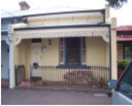
RICHMOND WALL STREET 14.jpg
