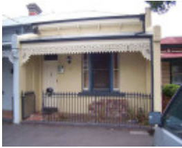
RICHMOND WALL STREET 14.jpg
