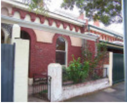
RICHMOND WALL STREET 35.jpg
