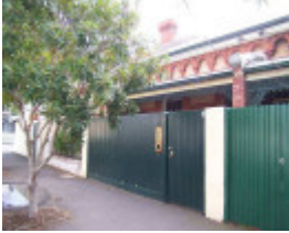
RICHMOND WALL STREET 37.jpg
