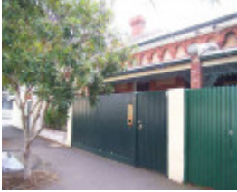
RICHMOND WALL STREET 37.jpg
