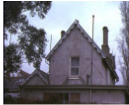
whitby house whitby street brunswick side view sep1979
