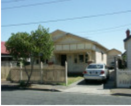
10a John Street, Geelong West
