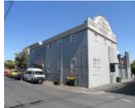
Former W James & Co Sack Merchants factory
