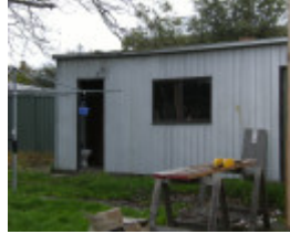
15 Lawton Avenue, Geelong West - Exterior Rear Shed
