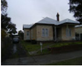
15 Lawton Avenue, Geelong West - Exterior Front View
