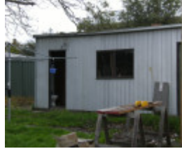
15 Lawton Avenue, Geelong West - Exterior Rear Shed
