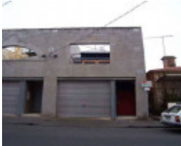
RICHMOND LYNDHURST STREET 52 Unit 1.jpg
