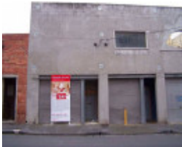
RICHMOND LYNDHURST STREET 52 Unit 4.jpg
