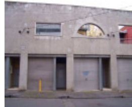
RICHMOND LYNDHURST STREET 52 Unit 3.jpg
