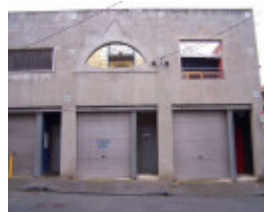
RICHMOND LYNDHURST STREET 52 Unit 2.jpg
