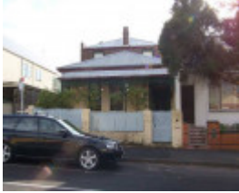
RICHMOND CHARLOTTE STREET 21.jpg
