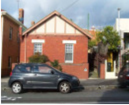
RICHMOND CHARLOTTE STREET 24.jpg
