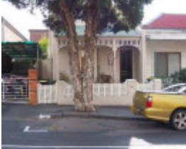
RICHMOND CHARLOTTE STREET 25.jpg
