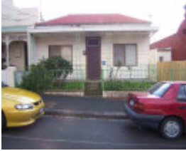
RICHMOND CHARLOTTE STREET 27.jpg
