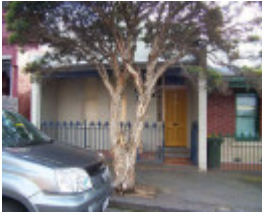
RICHMOND CHARLOTTE STREET 31.jpg
