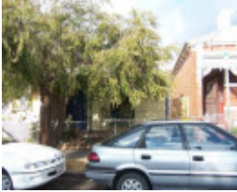
RICHMOND CHARLOTTE STREET 36.jpg
