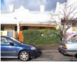
RICHMOND CHARLOTTE STREET 40.jpg
