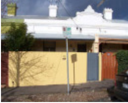
RICHMOND CHARLOTTE STREET 42.jpg
