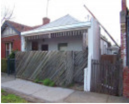
RICHMOND CHARLES STREET 71.jpg
