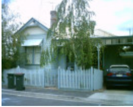
1 Lupton Street, Geelong West
