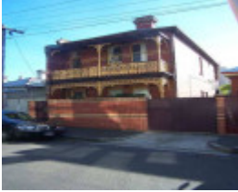
RICHMOND HULL STREET 9.jpg
