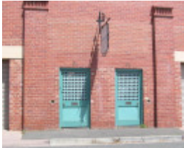
9a & 9b Lupton Street, Geelong West
