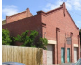
9a & 9b Lupton Street, Geelong West
