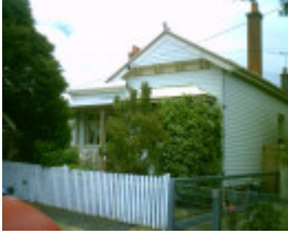
17 Lupton Street, Geelong West
