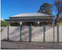
RICHMOND BANK STREET 8.jpg
