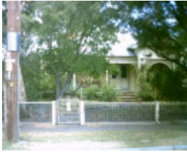
27 Lupton Street, Geelong West
