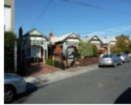
15-21 Bell Street, Richmond
