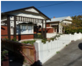
15-21 Bell Street, Richmond
