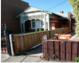
15-21 Bell Street, Richmond
