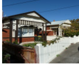
15-21 Bell Street, Richmond
