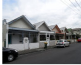
72-80 Stawell St from the south (no. 80 at far left)
