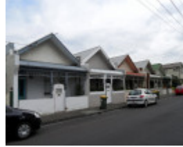
72-80 Stawell St from the south (no. 80 on the far left)
