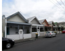
72-80 Stawell St from the south (no. 80 on the far left)
