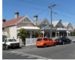
The houses viewed from the north (no. 85 at far right)
