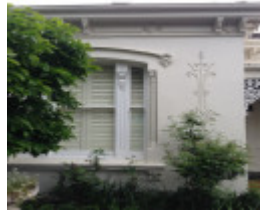
12 Newry St detail showing incised and moulded decoration to the projecting bay
