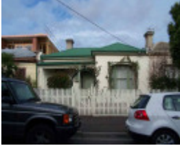
RICHMOND NEWRY STREET 14.jpg
