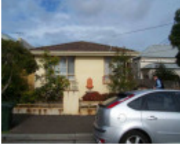
RICHMOND NEWRY STREET 20.jpg
