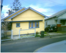
9 O'Connell Street , Geelong West
