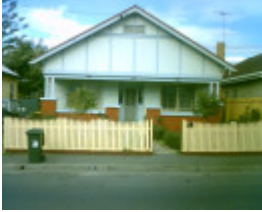
11 O'Connell Street, Geelong West
