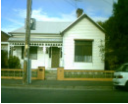
15 O'Connell Street, Geelong West
