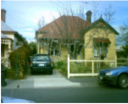
57 O'Connell Street Geelong West
