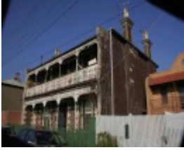
Richmond LESNEY STREET 20.jpg
